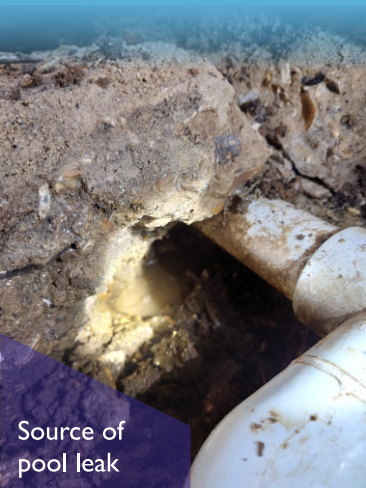
Source of pool leak and replacement pipework
